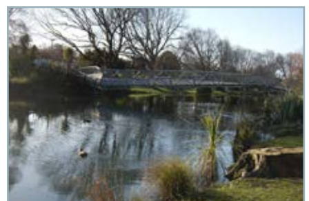
Twisted and damaged walk bridge
