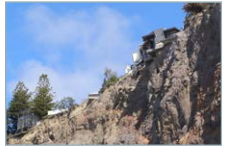
The houses - every one in danger
