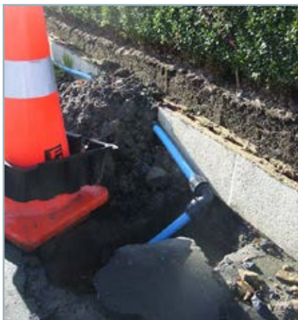
Above: typical street in bad areas - this was a bitumen road Below: Temporary water connection from the mains
