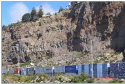
Shipping containers to protect the main road
