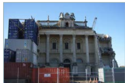
Severe damage to Catholic cathedral
