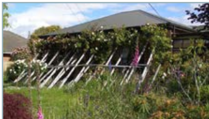
Supported walls of a house - a fruitless effort
