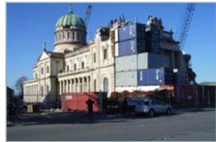
Catholic cathedral walls supported by shipping containers
