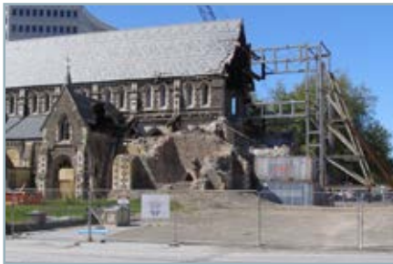
Cathedral damage, front and bell tower gone
